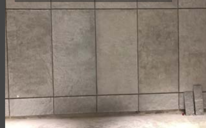
Installing Stone pattern
