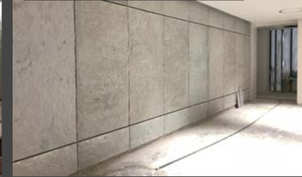
Installing Stone pattern
